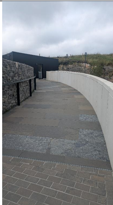
Ramp to Main Entrance from Disabled Parking Bays
