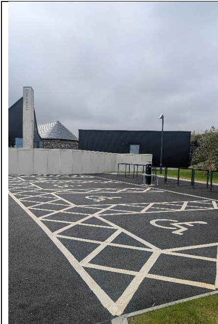
Disabled Parking Bays
